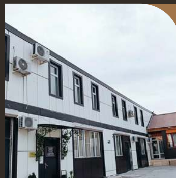
Eco House (Guest House)
